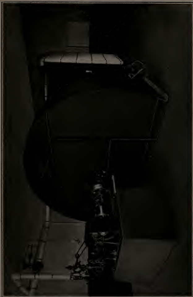
Fan, Heater and Engine Installation
